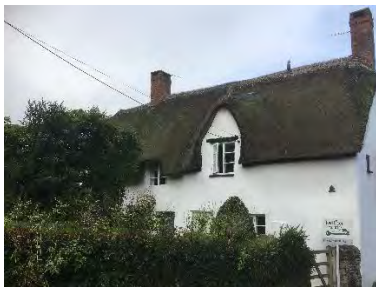
Cottage in Sea Lane, Kilve, BM
