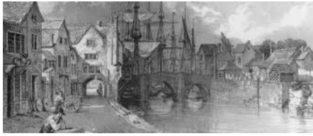
Old Bridgwater bridge
