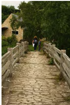
Tellisford packhorse bridge
