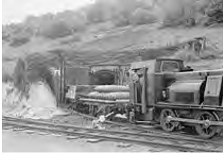
Railway to underground tunnels
